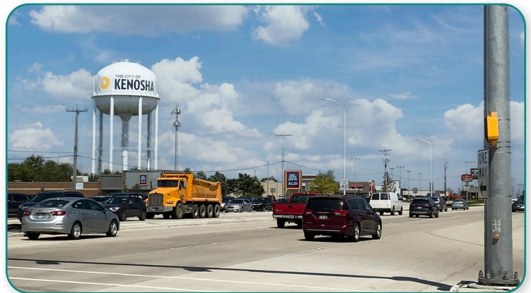
WIS 50 at Green Bay Road looking east
