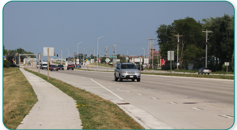
WIS 50 at 104th Avenue looking east
